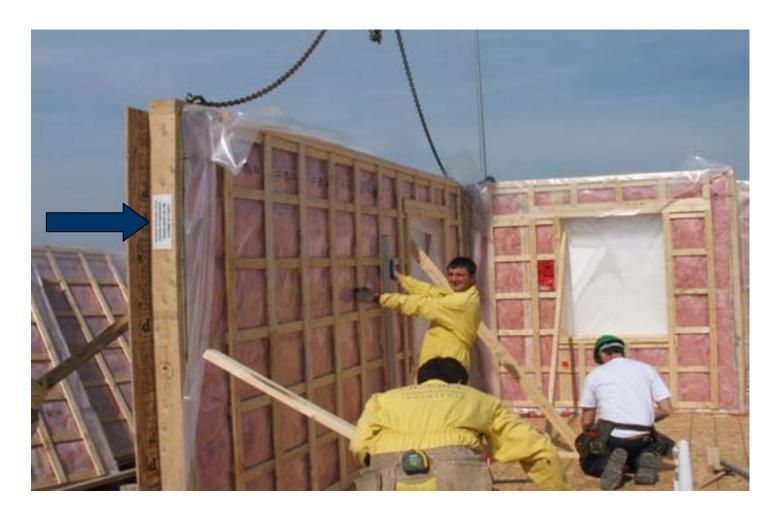
Note the label on the end of each panel detailing its instillation.
